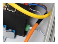
The connector has a white (5 V) and a black (GND) wire. When the module is mounted on the DIN rail, blue (5 V) is towards the bottom of the cabinet. The 5 V (white) cable is connected to the Support Module 5 V port (Pin 1 of the CAN connector). The black cable is connected to the power common GND distribution blocks of the DIN rail.
