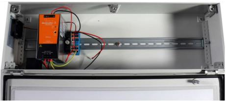
Figure 4.5: Control cabinet with Power Supply, without Modular Control Electronics.
